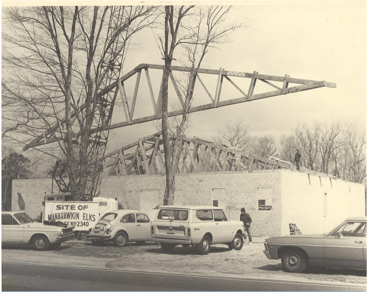
520 Hilliard Boulevard – New Building Construction 1970-1971
