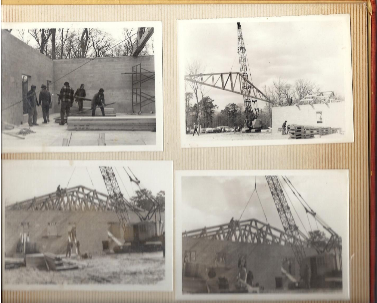
520 Hilliard Boulevard – New Building Construction
