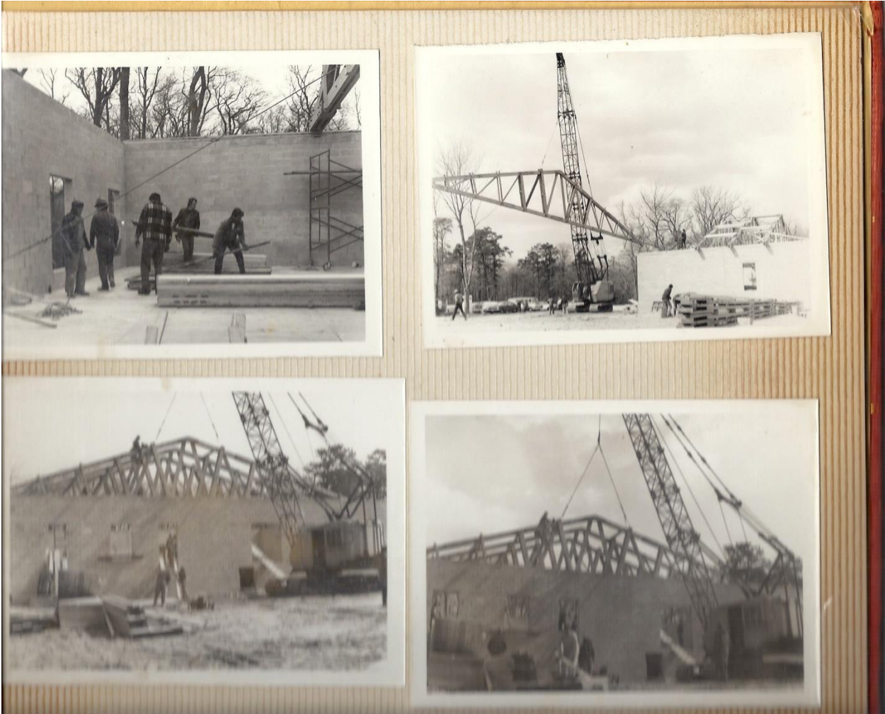
520 Hilliard Boulevard – New Building Construction
