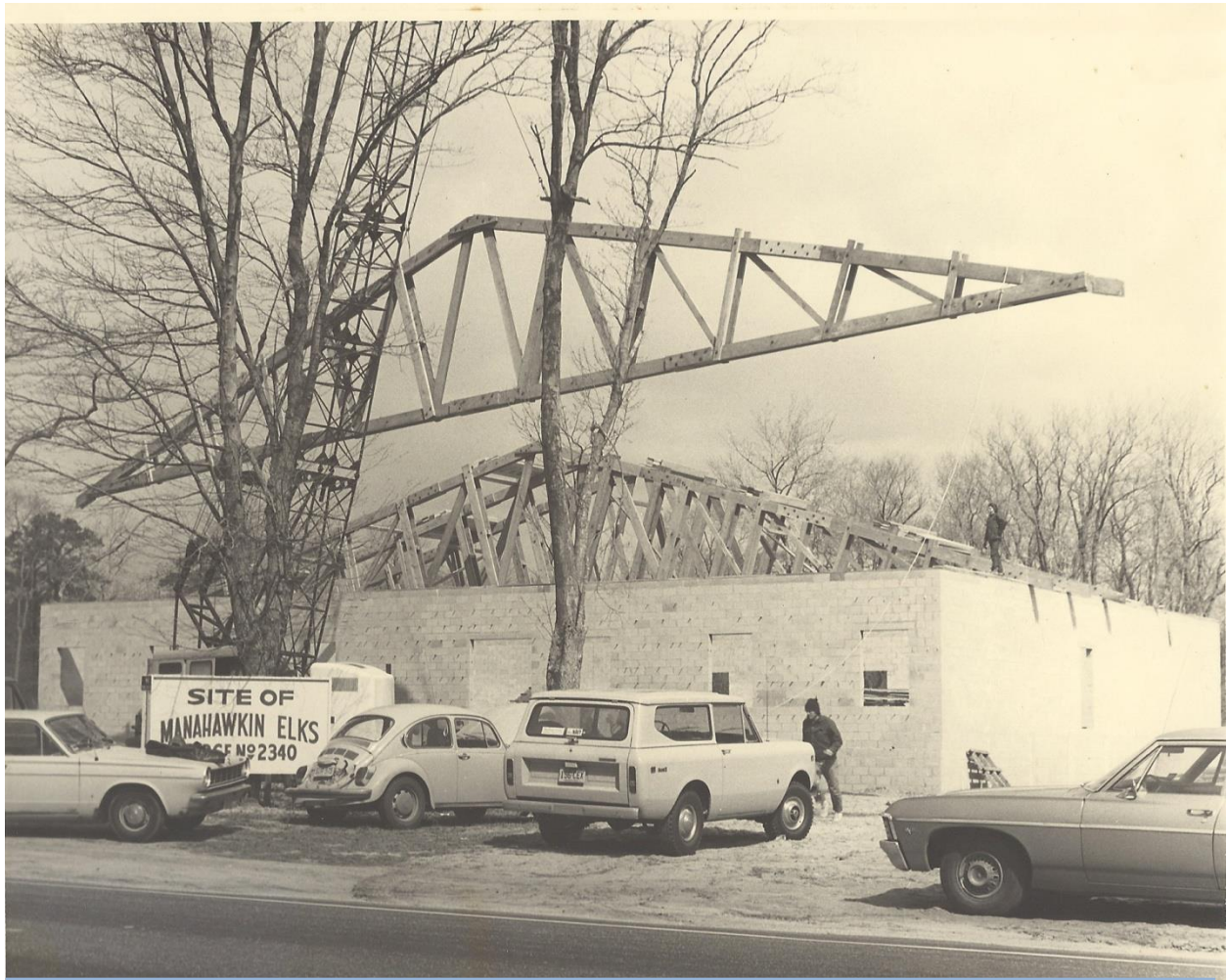
520 Hilliard Boulevard – New Building Construction 1970-1971
